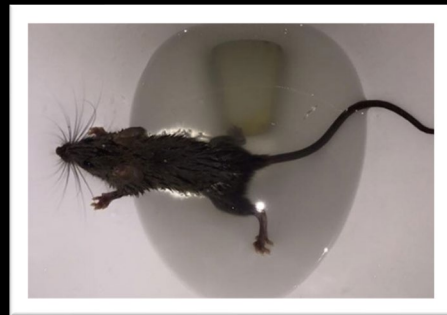
Figure 3: rat in toilet
